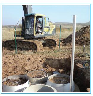
2008: 3-Channel Lysimeter station Friedrich-Schiller-Universität Jena: 1 x monolithic extracted lysimeter, 2 x filled lysimeters, gravity lysimeter.
