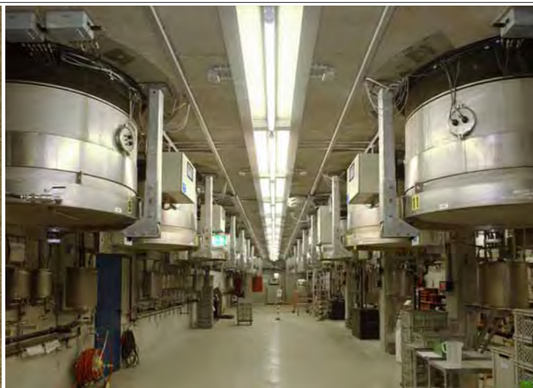
View of the service cellar
