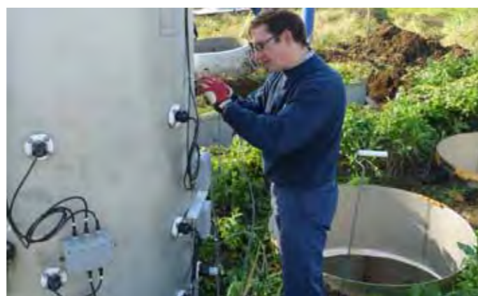
Inspection of the sensor installation
