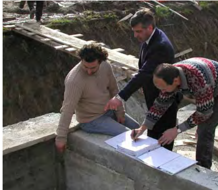
At the construction site
