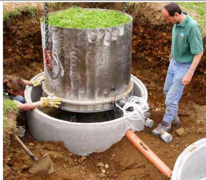
Installation of the Hydro-Lysimeter
