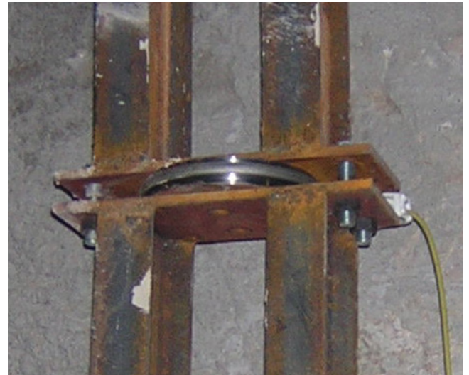
Load cell between two steel lining sections
