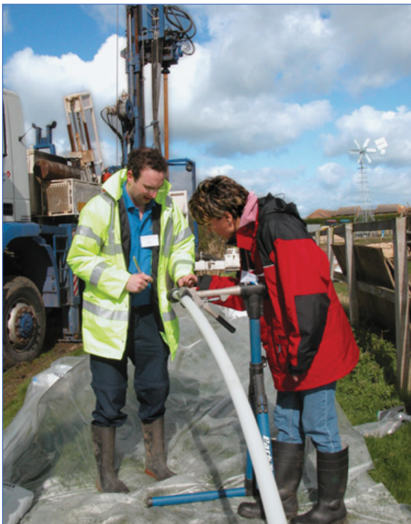
Construction of CMT ports in a 7-Channel System installed in Silsoe, England.
