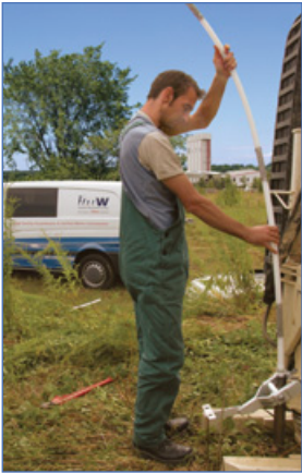
3-Channel CMT installation at a plant in Zeitz, Germany. Systems were completed using natural collapse and are being used to assess natural attenuation of BTEX.
