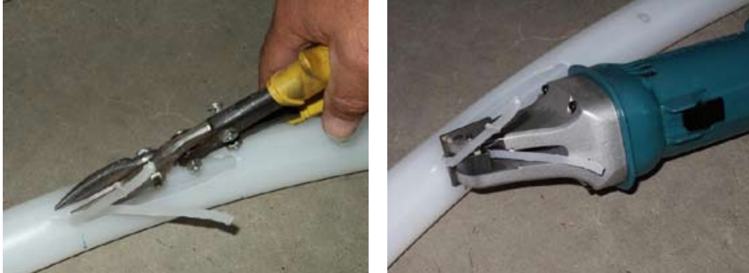
Fig. 10 Slotting the port
