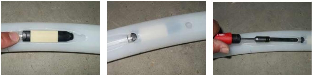
Fig. 11 Putting pie plug in place
