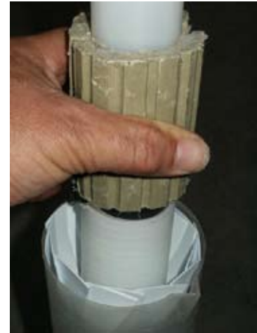
Fig. 18 Fitting BentoBlocks
