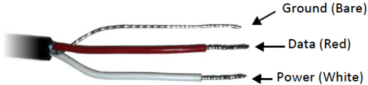
Figure 9: Pigtail End Wiring
